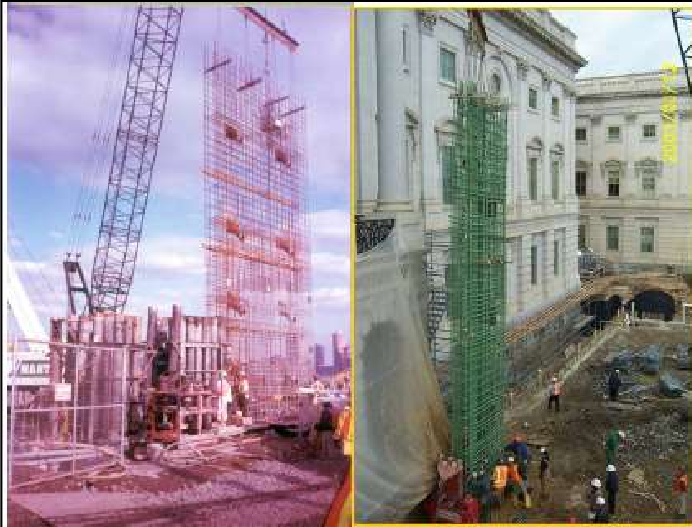
Cage Placement Note blockouts for floor slabs and trumpets for anchors .
